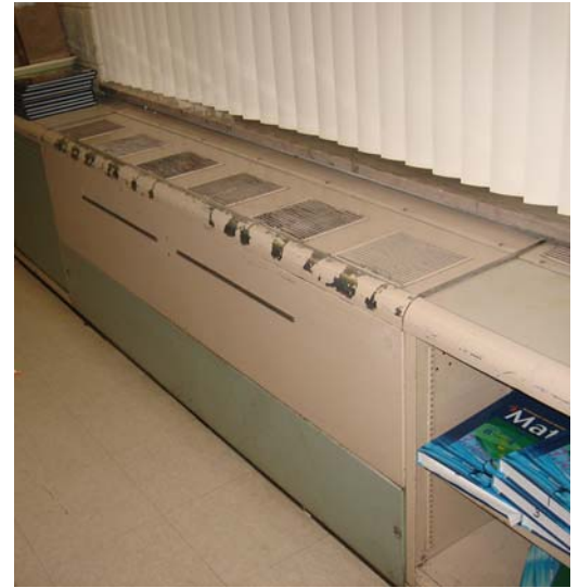
Existing Classroom Unit Ventilator and Heating & Ventilating Unit from the 1960s
