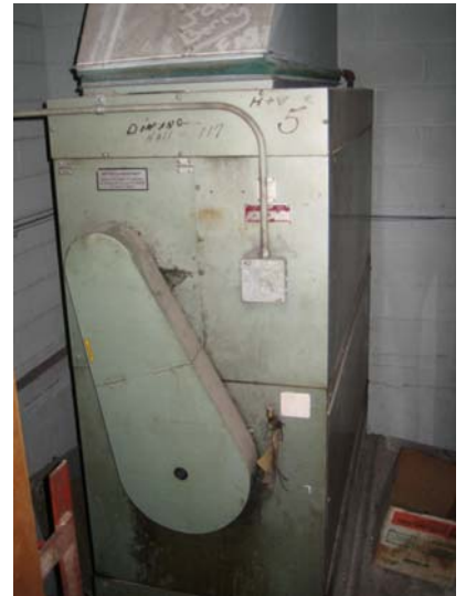
Existing Classroom Unit Ventilator and Heating & Ventilating Unit from the 1960s
